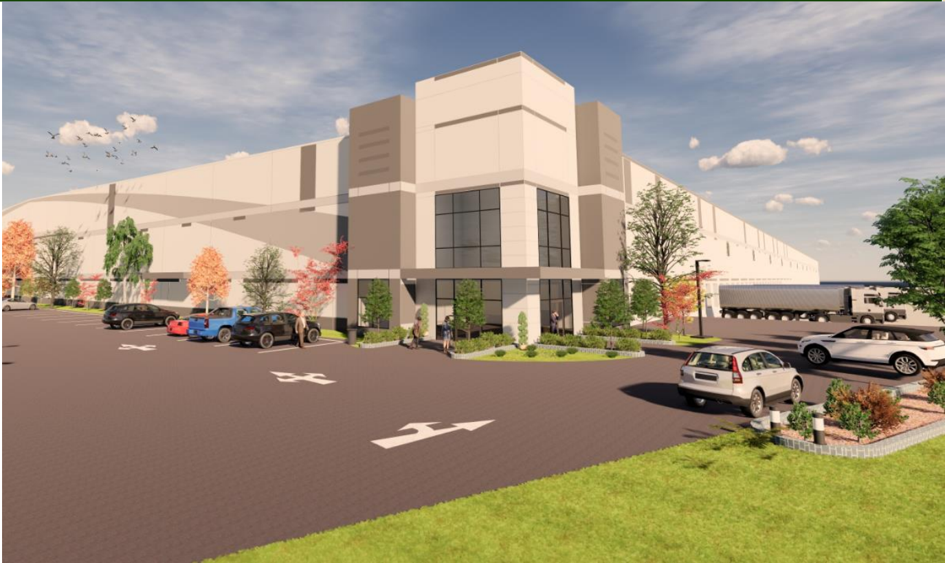
Artist's Rendering of Building under construction
