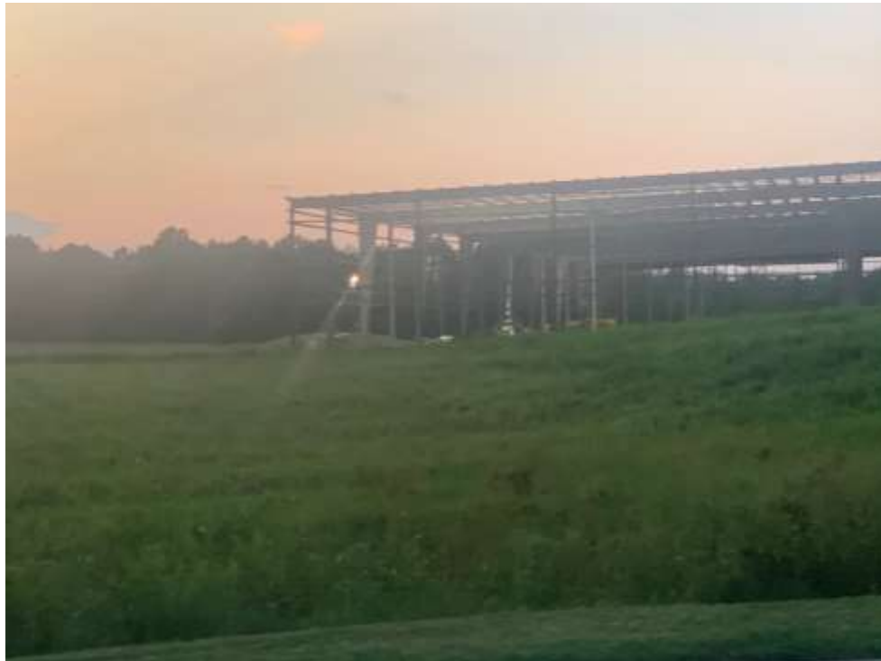
Property Photograph 14 – Building under construction, adjoining west
