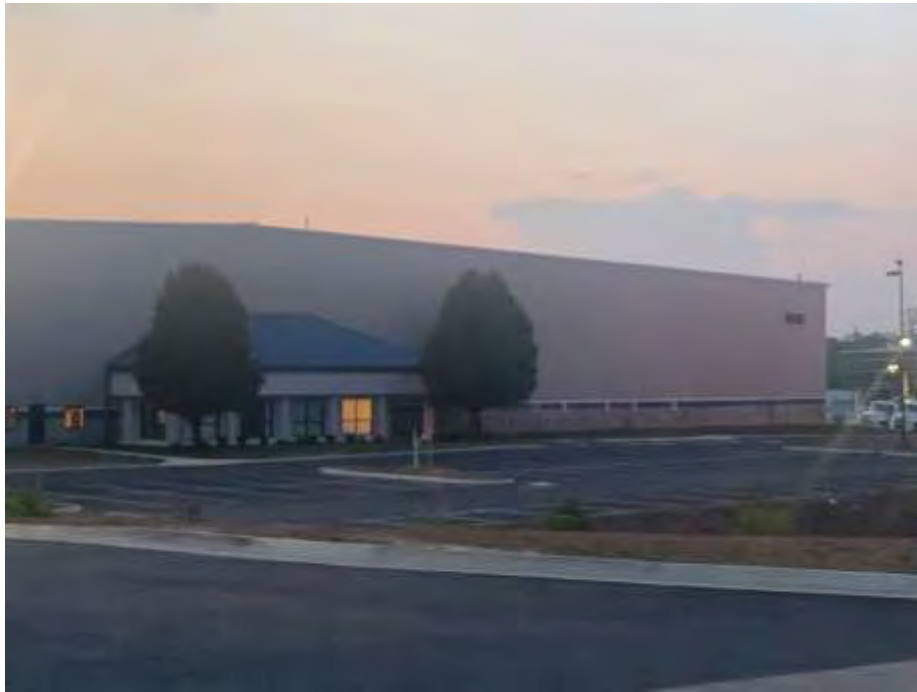
Property Photograph 13 – Diamond Plywood, adjoining west
